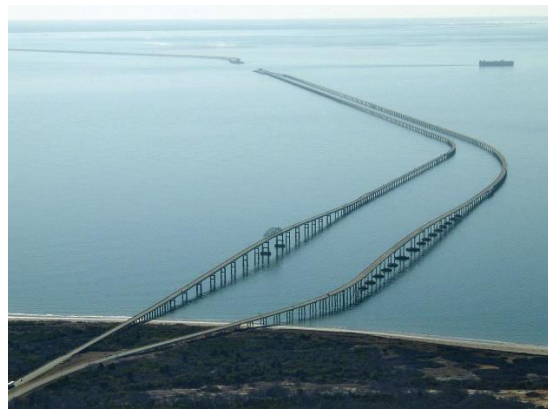
Chesapeake Bay Bridge-Tunnel
